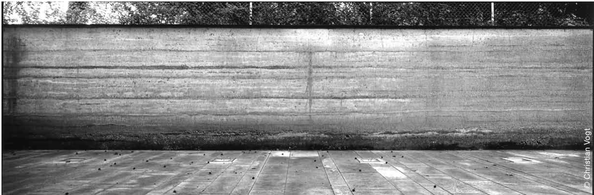
A wall made of rammed clay recalls a section cut into the soil showing various soil horizons and creating a colourful picture whose intensity varies with the weather. The fascinating mass of rammed clay and the pleasant climate it helps generate are quite noticeable on the terrace
